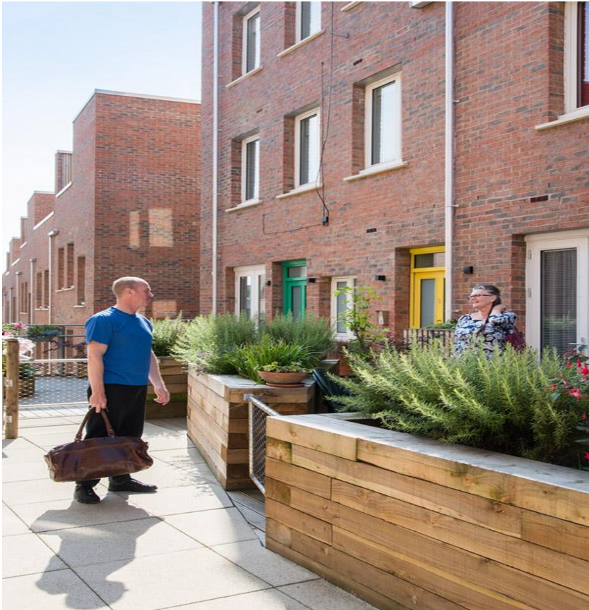
Figure 25: image showing small, enclosed gardens providing privacy to habitable rooms
